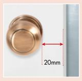
Minimum space 20mm between the doorknob and the start of the inner molding.
