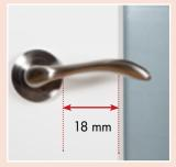
Minimumspace of 18mm between the doorknob and the start of the inner edge of the molding.
